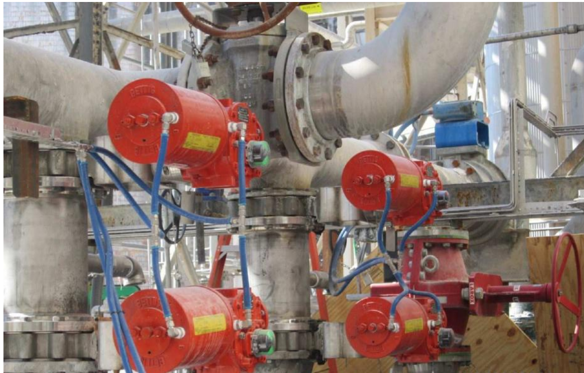
Tricentric white liquor lime mud pump isolation
